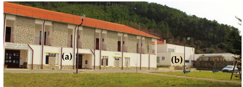
Social and Cultural Center of Santo Aleixo: (a) residential building; (b) building of new valences.
