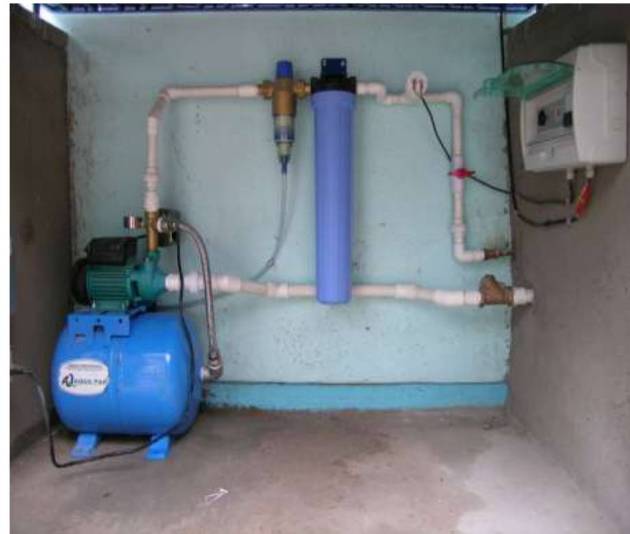
Pump and basic filtration system. Solar-powered Silver Ionizer to the right
