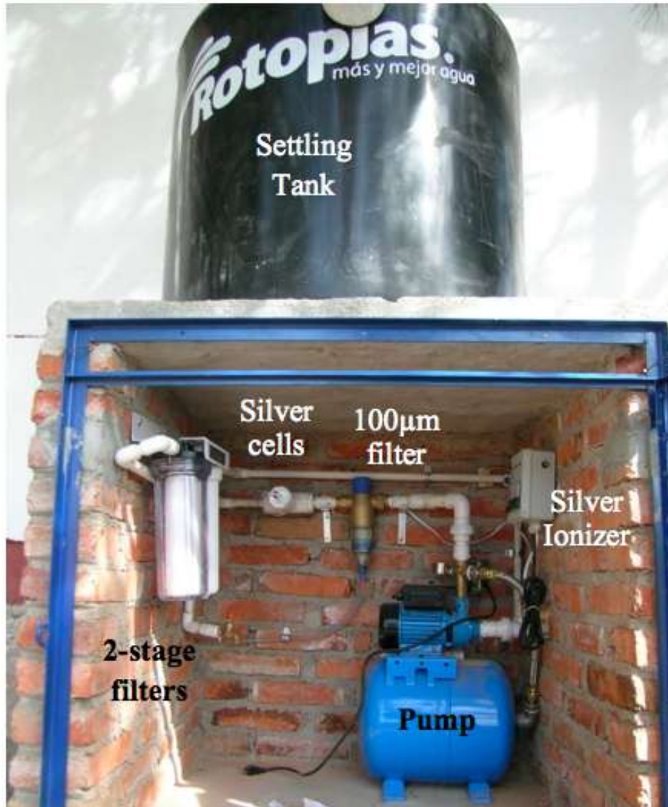
Pump and basic filtration system. Solar-powered Silver Ionizer to the right
